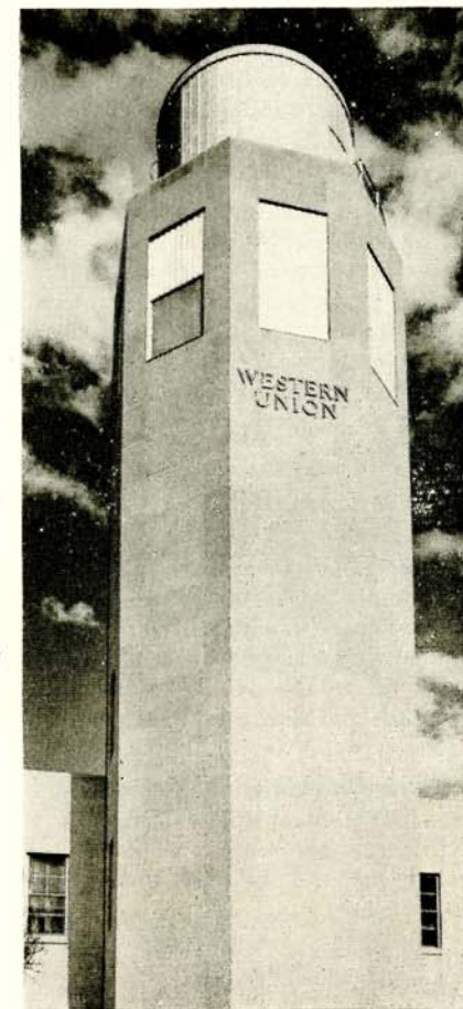
The radio relay tower at Washington, D. C. Note the fibre-glass windows which are used to protect the reflectors.
