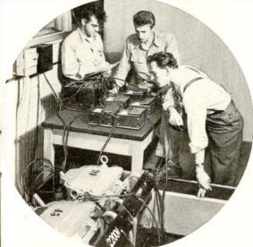
This experiment in the electrical laboratories is being performed by students to determine the characteristics of a 2,200 volt transmission line. Readings are recorded and used in completing requirements for class reports. Career Note: Without power, none of the major advances in science, construction, industry or business would have been possible.
