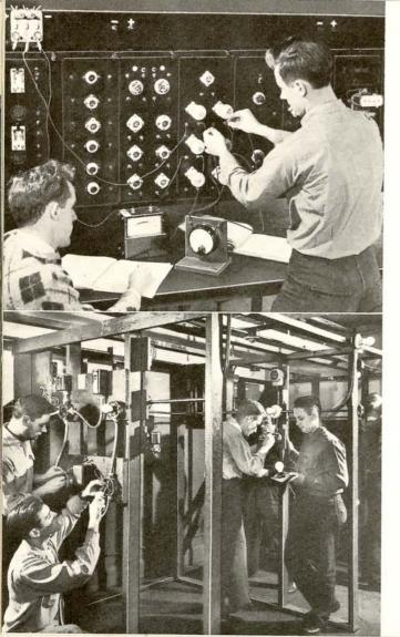
Practical experience gained during the first terms provide a foundation upon which students are able to understand the theoretical training of advanced electricity. Here students are using a unit test board to determine measurements of resistance in series and in parallel. Career Note: Electricity, harnessed and put to work in a multitude of ways, has changed - and made more attractive - the face of civilization. Despite a half century of progress, its development has just begun.
