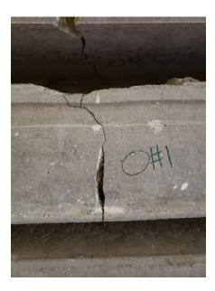
Figure E- 29. Offset #1 side cracks.
