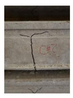
Figure E- 15. Center #2 side cracks.
