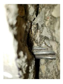
Figure E- 7. Center #1 exposed strand in crack.
