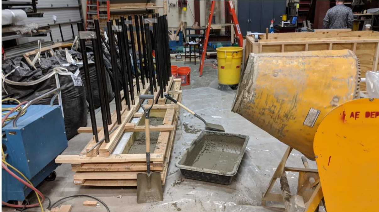
Figure 15 – 2 nd Concrete Pour Day.
