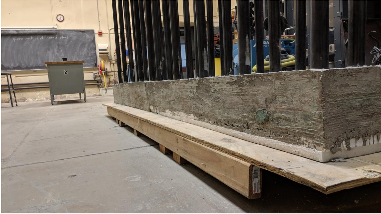
Figure 19 – Concrete Members with Form Walls Stripped.
