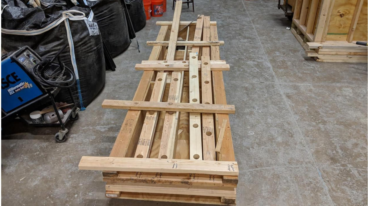
Figure 14 – Empty Concrete Form.
