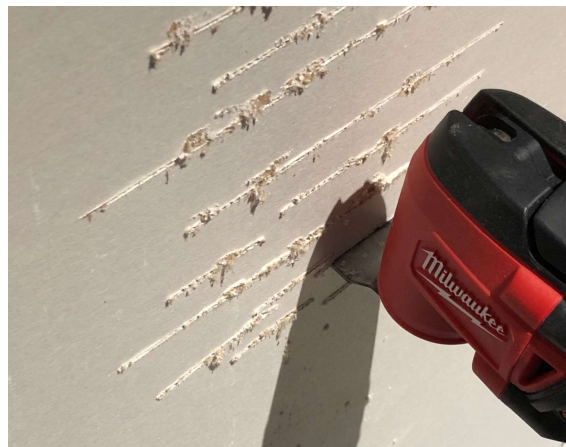
Figure 62: Plunge Cutting Drywall.
