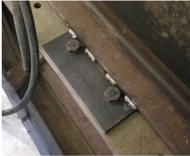
Figure 3.5.1-1. Welded connection of steel channel to base plate.
