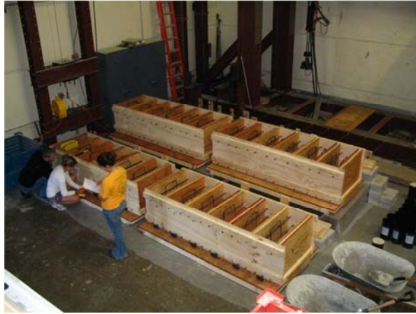
Figure 24 – Typical Formwork [2].
